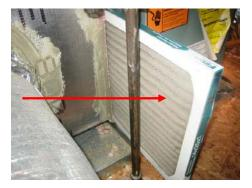
FYI: The filter size for both HVAC units is 14" x 25" x 1." The filters should be replaced at least once every three months.
