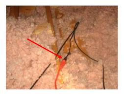
A duct in the Attic serving the Second Floor Hallway Bathroom exhaust vent has several holes that appear to be the result of a rodent (SEE PHOTO). Recommend replacement of damaged exhaust vent duct in Attic and evaluation and treatment if necessary by a qualified pest control technician.
