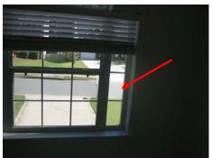
Deformed spacer seals are noted at the sidelight windows at the front entrance (SEE PHOTOS). This condition is the result of a manufacturing defect that causes the seals to expand when exposed to the heat of the sun. Recommend replacement of sidelights at front entrance.
